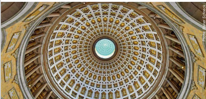
View of the dome with the glass lantern
